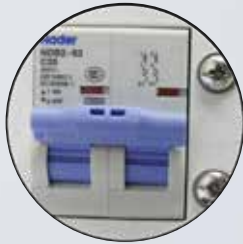
Electrical safety breaker
